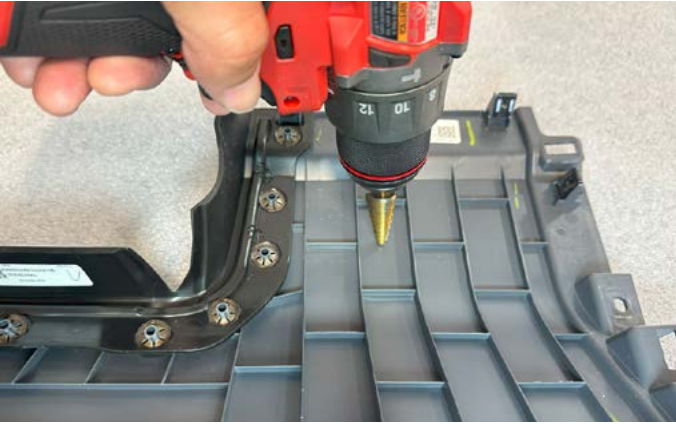
32. Mark your switch location and then use a unibit step bit to drill a 3/4" hole. Install switch into the panel. Use a 7/8" socket/wrench to tighten the switch nut.
