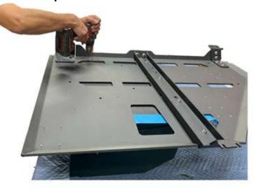
8. Place your box face down and then place the RDO plate assembly over box. Use the masking tape as reference for final box location. Locate the pre-drilled holes on RDO plate that best match your box. Use an 1/8" drill bit and drill the mounting holes into your box. Remove RDO plate assembly and drill 1/8" holes to 3/8".
